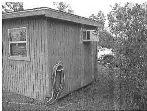
Rear Face, North View
